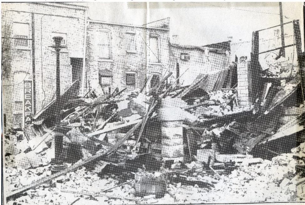
The breakfast sign and the lamppost stand intact in the remains of The Carlton.
