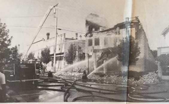
Many different streams of water are aimed from Henry Street at the smoldering remains of The Carlton.
